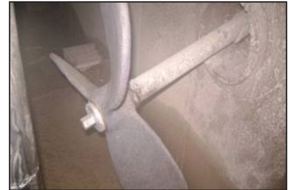
Completed agitator installed in tank
